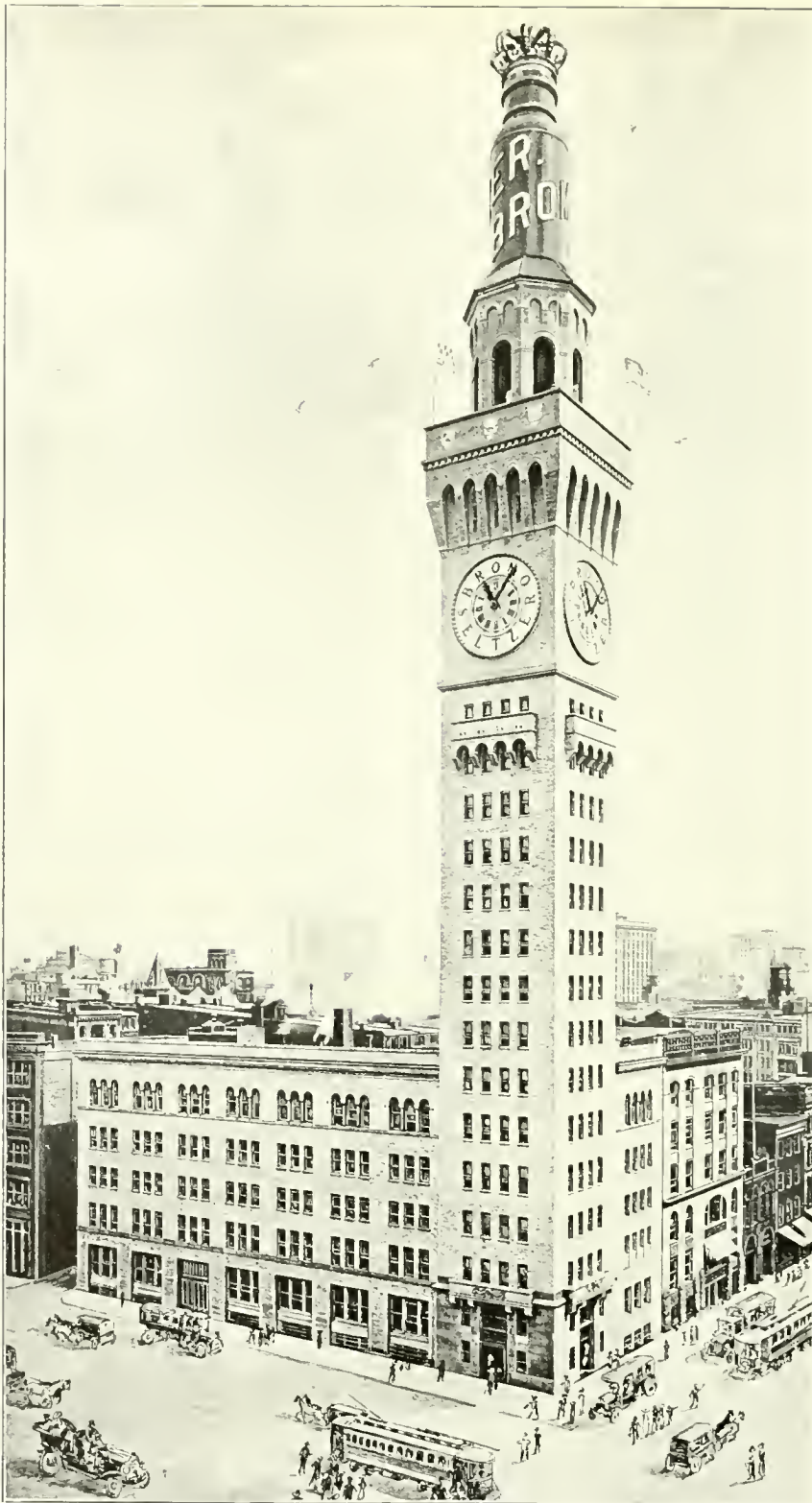
BROMO-SELTZER TOWER. Total height of tower, 357 feet. The Bottle on top, a fac-simile of the regular ten-cent Bromo-Seltzer bottle, but about 10,000,000 times larger, is 51 feet high, 20½ feet in diameter, weighs 17 tons, and revolves at the rate of 10½ feet per minute. There are 596 electric lights in bottle and crown surmounting it, which can be seen at a distance of 20 miles. The Bromo-Seltzer clock is the largest four-dial gravity clock in the world. The dial is 24 feet in diameter. The minute hand is 12 feet 7 inches long and weighs 175 pounds. The hour hand is 9 feet 8 inches long and weighs 145 pounds. The pendulum is 35 feet long and weighs 475 pounds. The clock is automatically wound by an electric motor every six hours.
